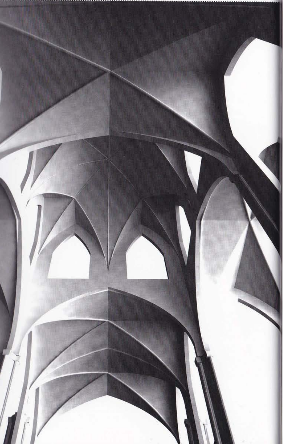
The nave of the Church of Our Dear Lady is formed by the horizontal tessellation of a series of cross-vault base units that are repeated along the length of the nave. Changes in the arrangement of the base units in plan, from linear in the center to curved along the edges, vary the profile of the nave to give it a mostly rounded plan. Changes in height between the nave and the side aisles allow for the introduction of openings along the elevation. The nave of the Church of Our Dear Lady transmits an optical affect of roundness, verticality, symmetry and crystallinity, and an acoustical affect of diffusion and slowness.
